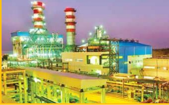
225 MW Sikalaha Combined Cycle Power Plant, Bangladesh
