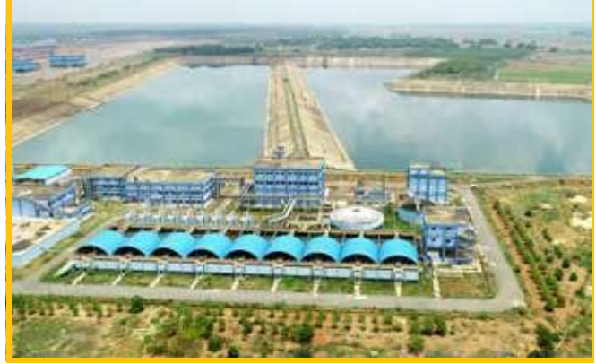
NMDC WTP & Reservoir, Chattisgarh
