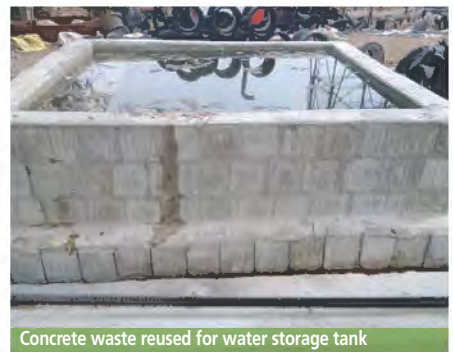
Concrete waste reused for water storage tank
