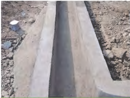
Concrete waste reused to create drains
